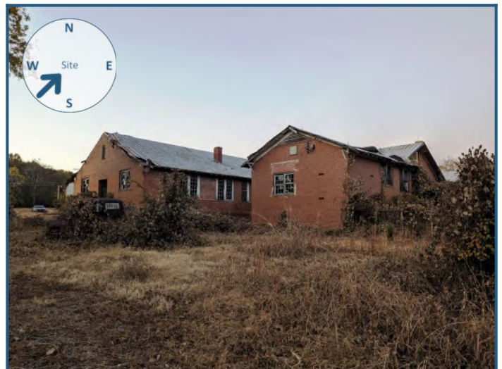
View of site from the southwest
